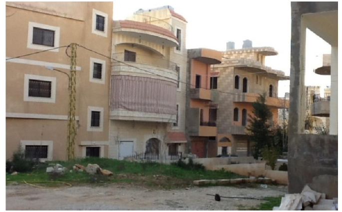
Figure 2. Old Town of Bint Jbeil after reconstruction
