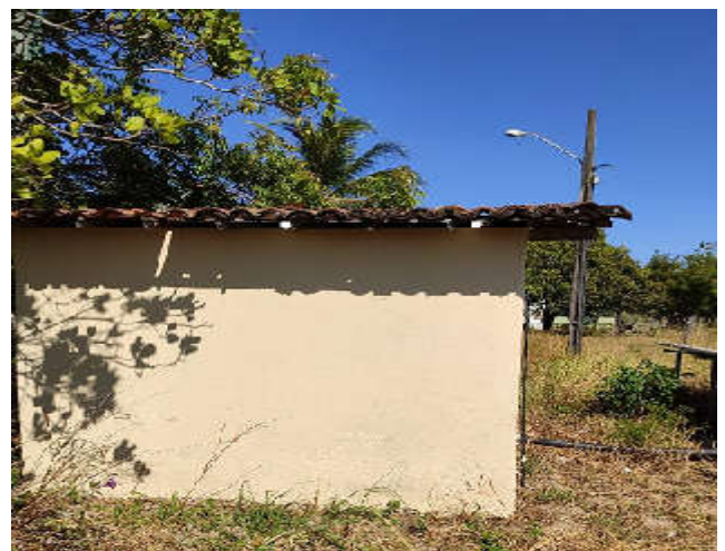
Fig. 4. Masonry room where the electrical structure was built
