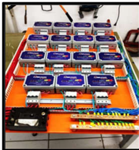
Figure 13. Panel with the 15 Capacitive Filters Assembled for application in the QGBT/220V
