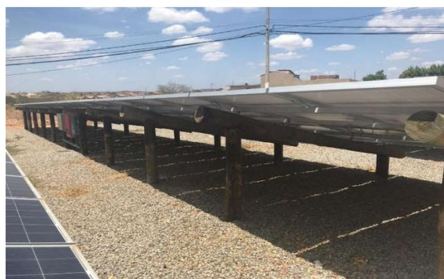
Figure 4. Base with eucalyptus for support of photovoltaic modules
