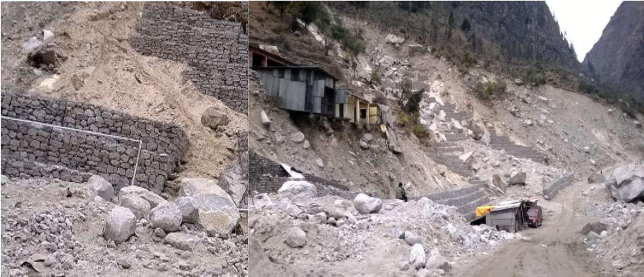
**Plate 13. Inappropriate construction of retaining walls on Badrinath road near Lambagad GP**
