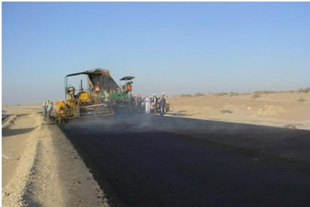
**Figure 4. Fumes released from behind the paver**
