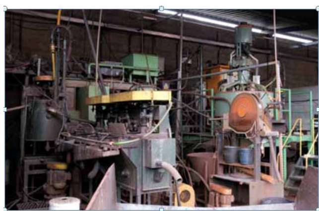
Fig. 6. Adjustable plant used for testing in Gorceix Foundation (Souza et al., 2016)
